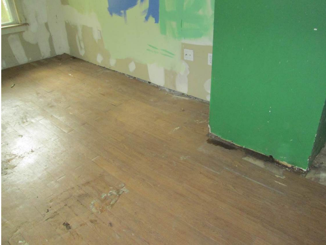
Dining Room floor showing separation from chimney flue.
