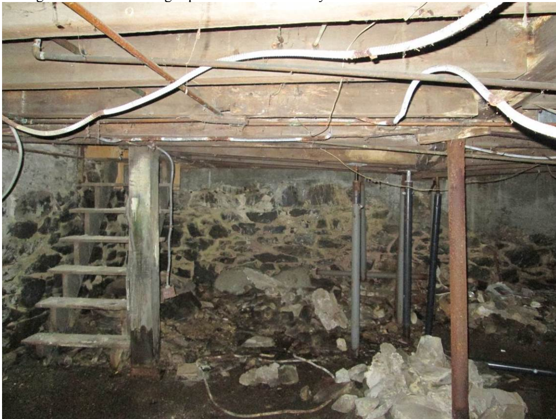
Basement showing lally columns beneath dining room area.
